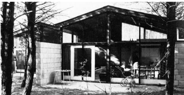
Sporthuis Centrum, vacation houses Lommerbergen (exterior view), 1966
